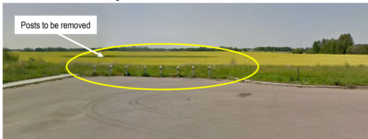
Figure 27 - 49 Ave / Westview Drive Post Removal - Looking West
