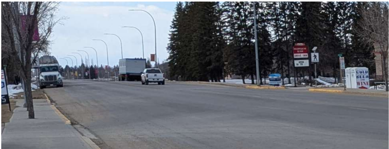
Figure 7.2: Example of an Urban Roadway in Calmar - 50 Avenue (Source: ISL)
