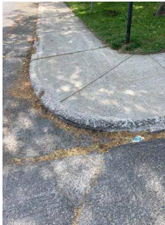
Missing Wheelchair Ramps
