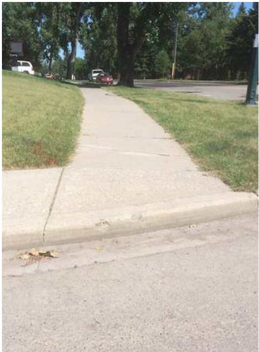
Missing Wheelchair Ramps
