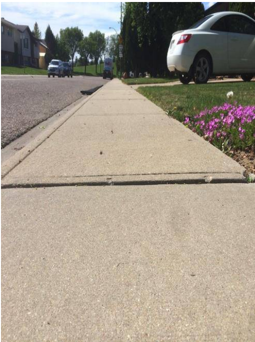
PRV 1 Vertical Displacement
