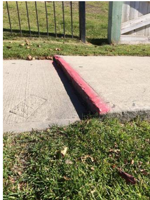
PRV 3 Vertical Displacement
